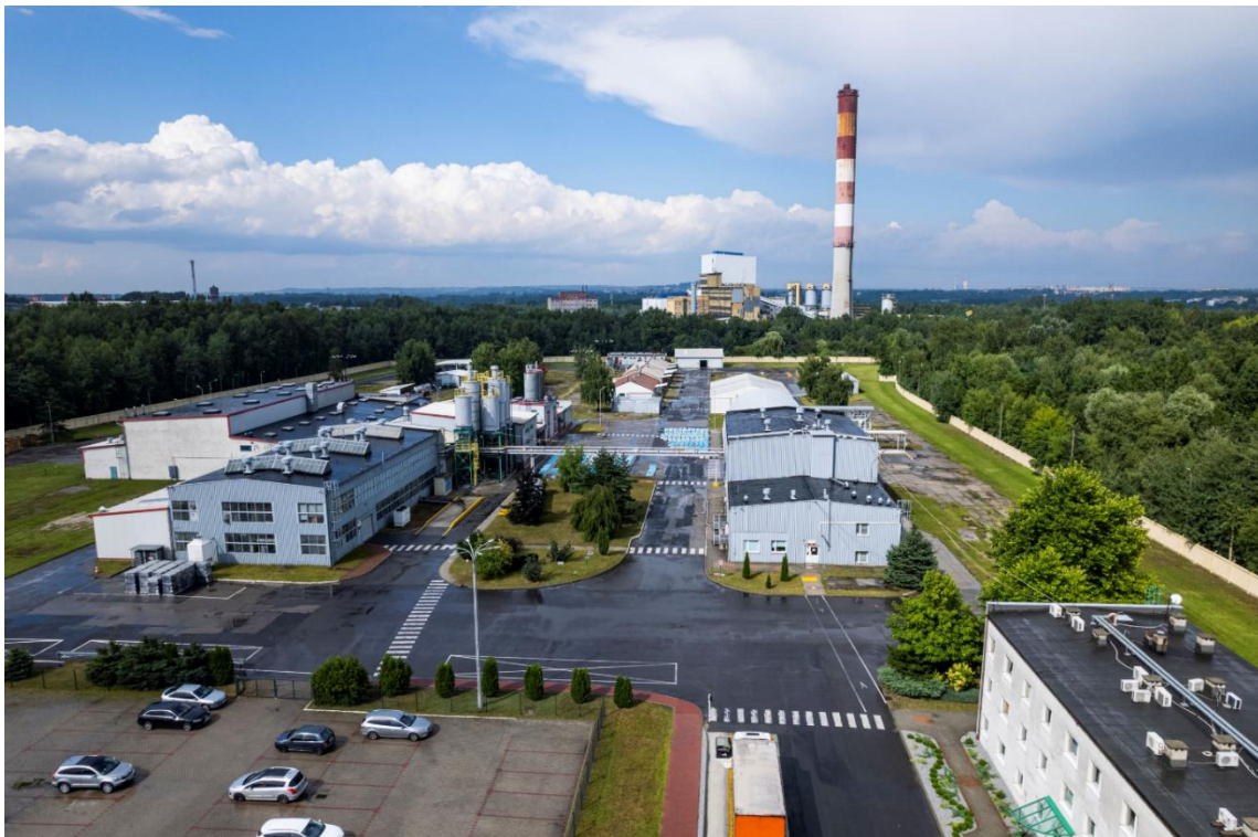
Fig. 1. A view of the MINOVA EKOCHYM Sp. z o. o. production plant located in Siemianowice Śląskie (Poland)
