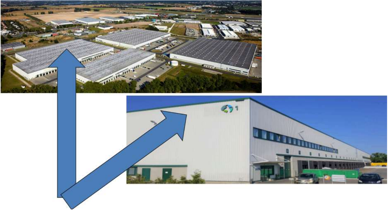
Fig. 1. IBP Instal fittings plant at ul. Za Motelem 2A in Sady/Tarnowo Podgórne (Poland)
