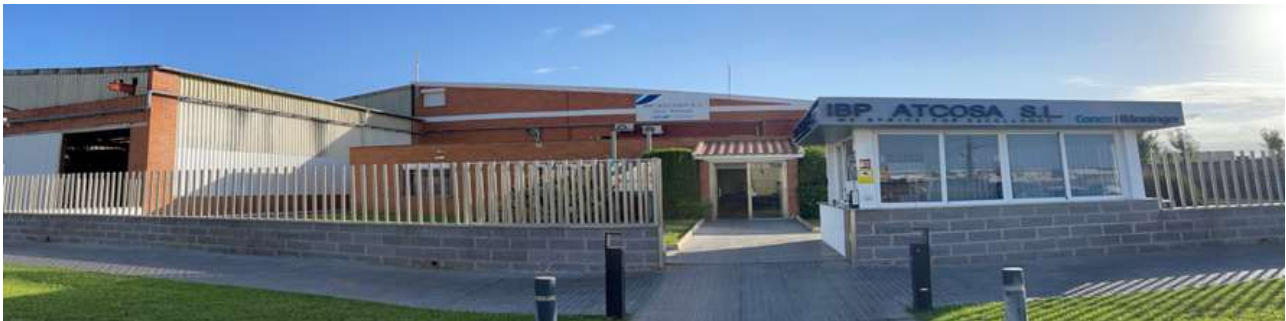
Fig. 2. IBP ATCOSA plant, Poligono Industrial, Quintos-Aeropuerto in Cordoba (Spain)
