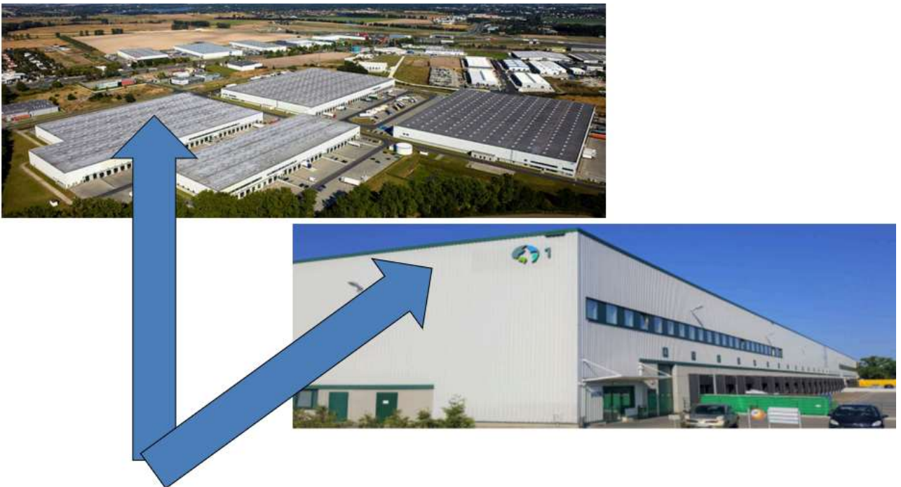
Fig. 2. IBP Instal fittings plant at ul. Za Motelem 2A in Sady/Tarnów Podgórny (Poland)
