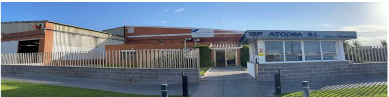
Fig. 3. IBP ATCOSA plant, Poligono Industrial, Quintos-Aeropuerto in Cordoba (Spain)
