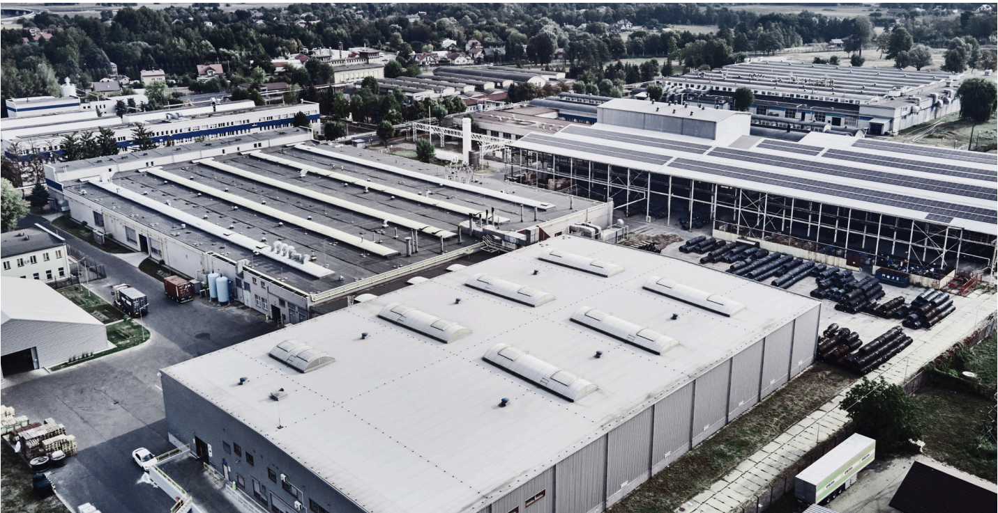
Figure 1. Manufacturing plant view
