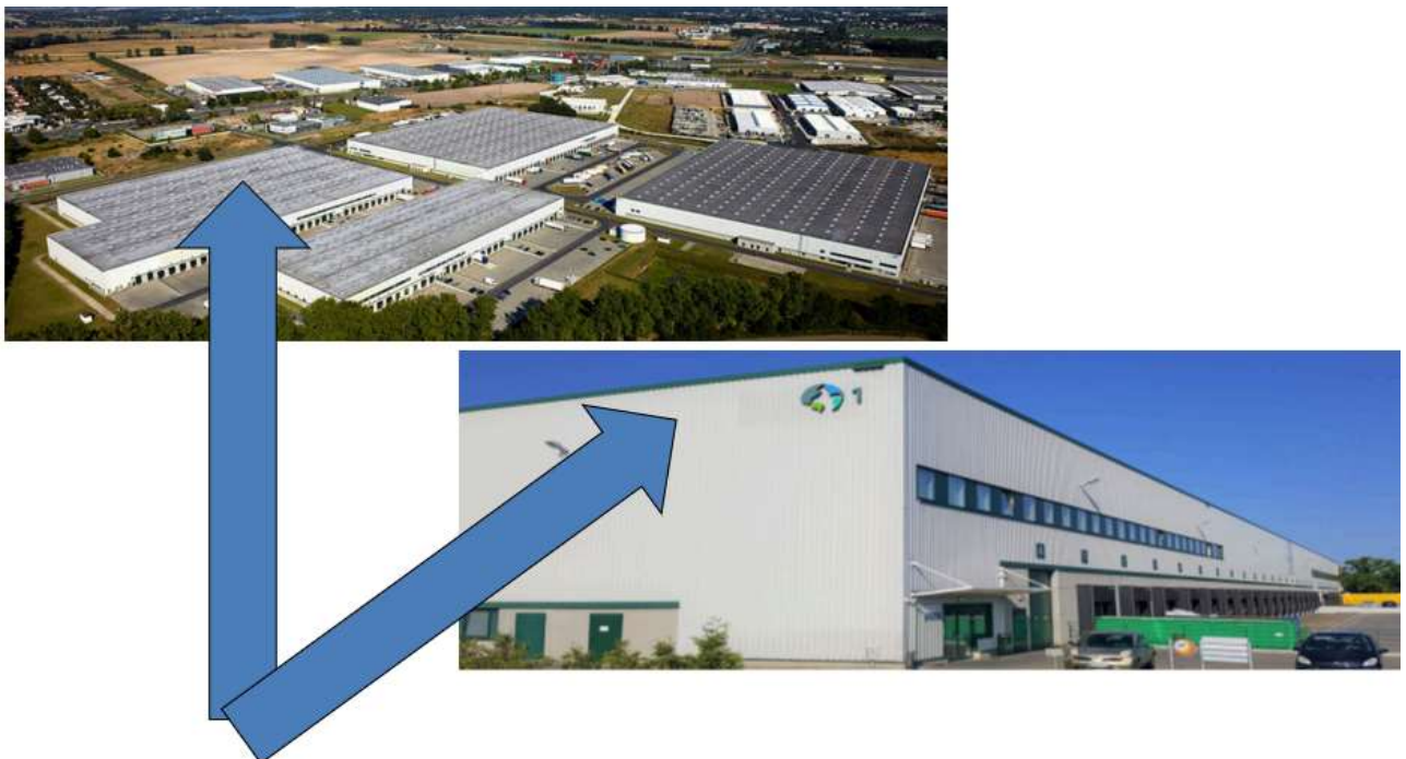
Fig. 2. IBP Instal fittings plant at Za Motelem Street 2A in Sady/Tarnów Podgórny (Poland)
