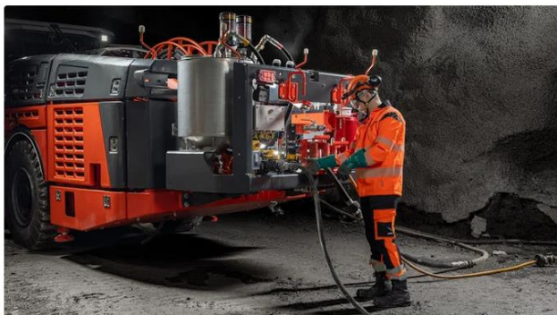
Fig. 2. Injection silicate resins in tunneling (left) and mining (right) operations.
