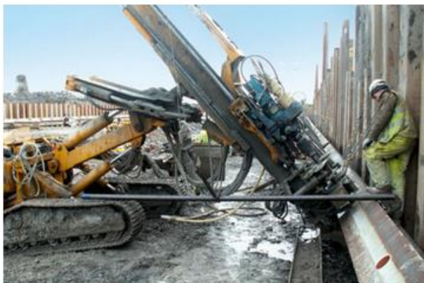
Fig. 2. Application operations of injection polyurethane resins.
