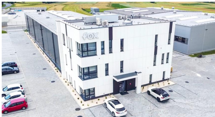
Figure 1 Street view of FOX FITTINGS Sp. z o. o.
