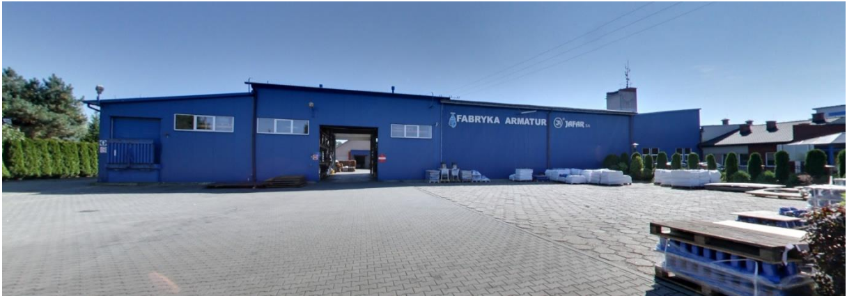
Figure 1 Street view of Fabryka Armatur JAFAR S.A.
